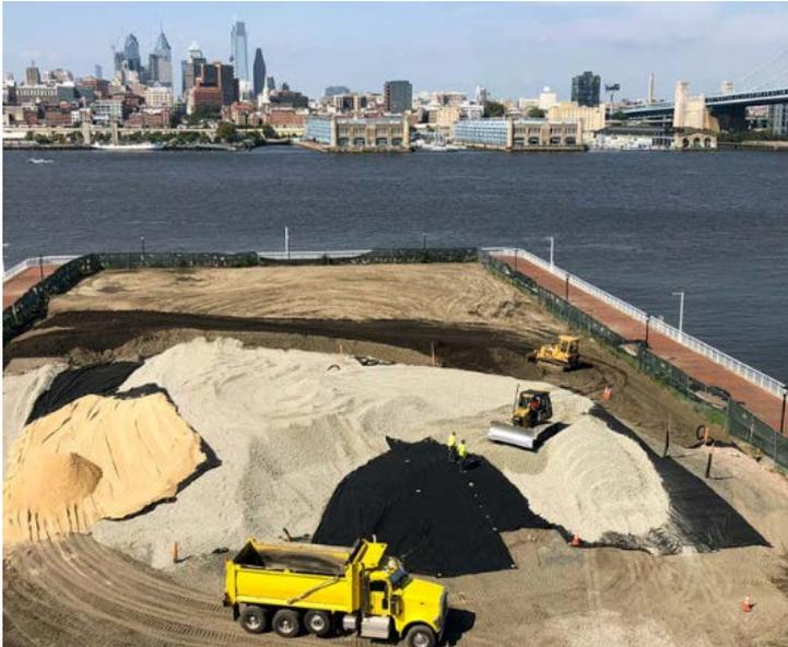
AeroAggregates is revitalizing local manufacturing and developing a circular solution for post-consumer recycled glass in the Philadelphia region. Their product, an ultra-lightweight aggregate called foamed glass, has applications in transportation, infrastructure and construction. AeroAggregates is the first vertically-integrated company in the United States to produce this product, which has been in use for several decades in Europe.
