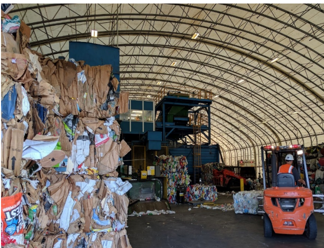
Figure 1. ECUA's MRF is a 53,000 square foot fabric and metal structure, which reduced the cost and construction time of the facility.
